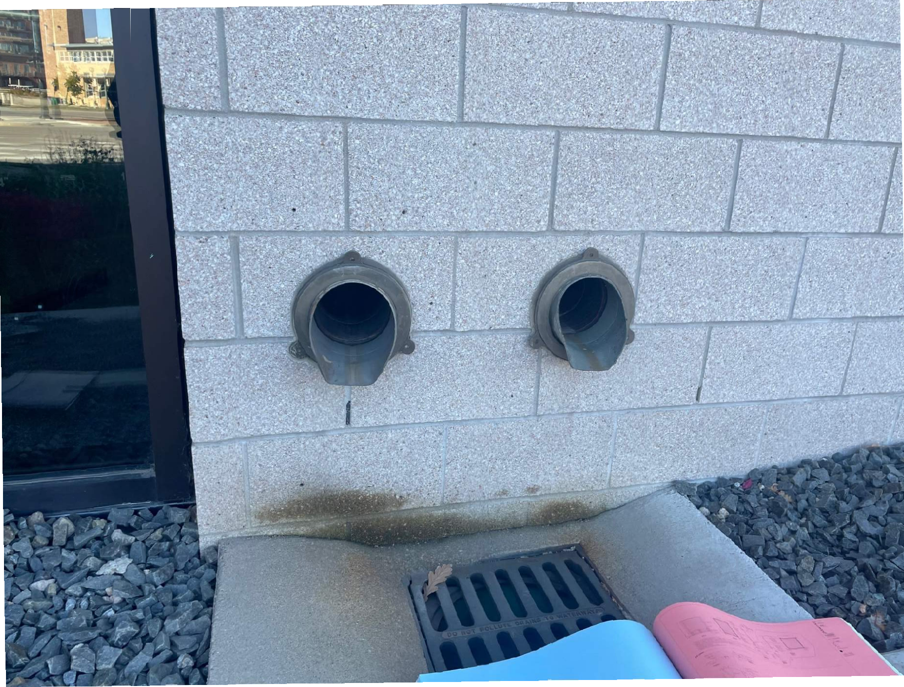
EXISTING ROOF DRAIN TERMINATIONS
