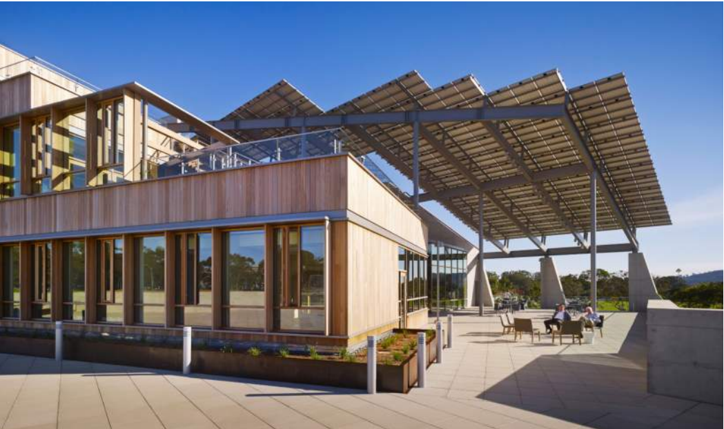
(Left) The J. Craig Venter Institute has two photovoltaic arrays comprising 26,124 SF of surface area that are predicted to exceed the building demand, pushing excess power generated back into the grid. These arrays are utilized as shading devices in most of the exterior spaces.
