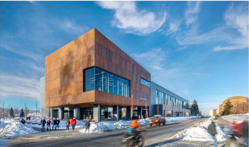
(Above) Rocky Mountain Institute Innovation Center utilized Factor 10 Engineering to further each sustainable strategy. The enhanced exterior envelope had a 4 year payback when considering it helped eliminate traditional mechanical systems and improved indoor environment quality resulting in increased productivity and engagement.
