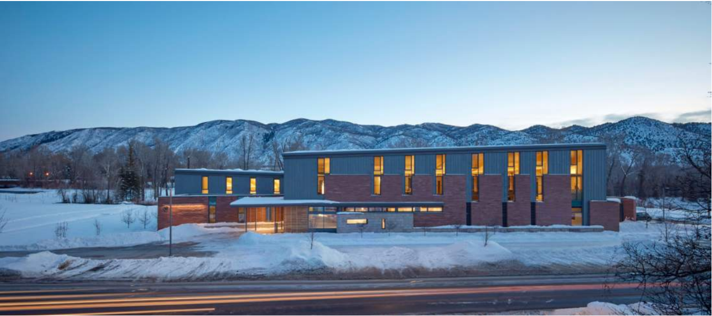
(Above) Rocky Mountain Institute Innovation Center utilized Factor 10 Engineering to further each sustainable strategy. The enhanced exterior envelope had a 4 year payback when considering it helped eliminate traditional mechanical systems and improved indoor environment quality resulting in increased productivity and engagement.
