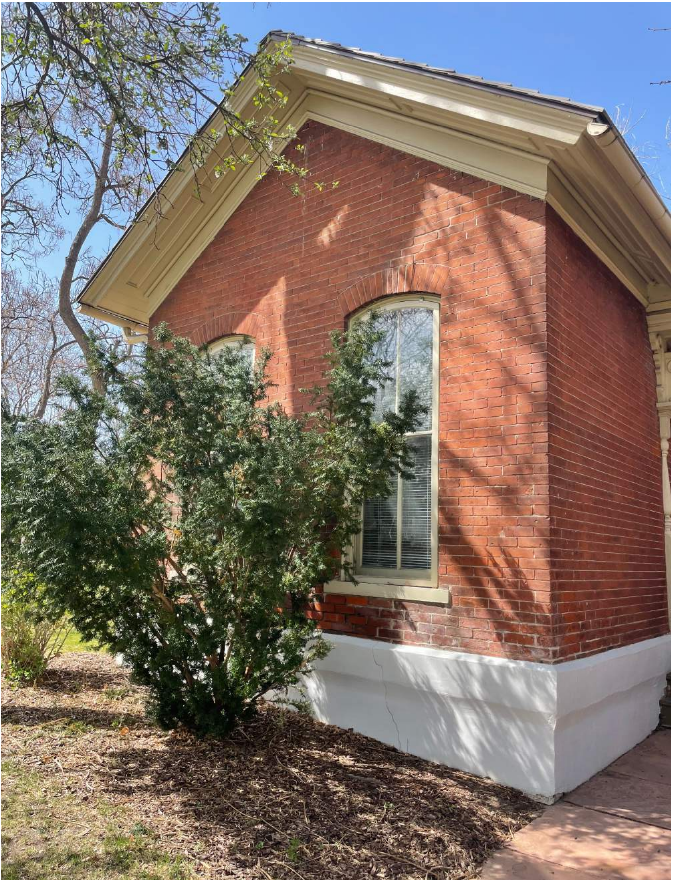
East facade with red brick walls, wood arched-top windows, parged foundation wall.
