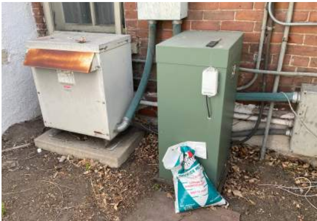
Transformer below the window mounted to a concrete pad serving the electrical wall panel. Rain bird irrigation system.
