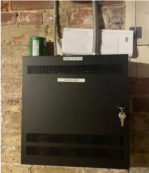
Fire alarm panel at north wall of Basement.
