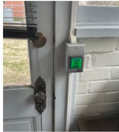
Push to exit hardware in existing Break Room.
