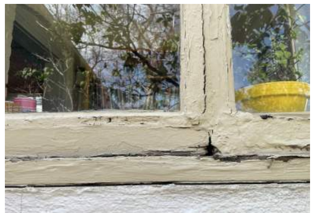
Deterioration of the wood window and sill at the north elevation of the rear addition.
