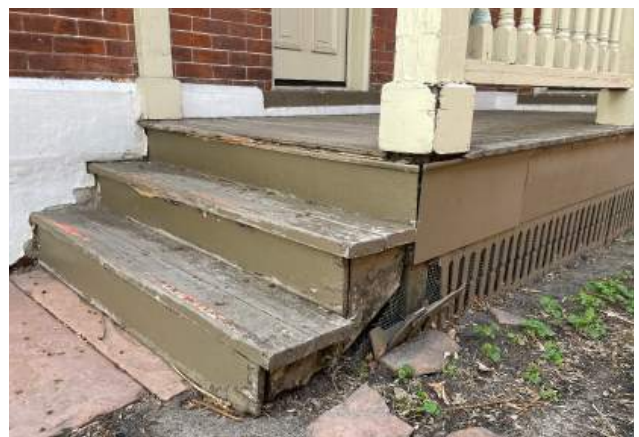
Wood stringer, floor structure, and screening material.
