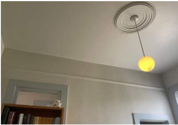
East wall and ceiling in existing Office 2. Non-original globe light fixture with plaster mold.
