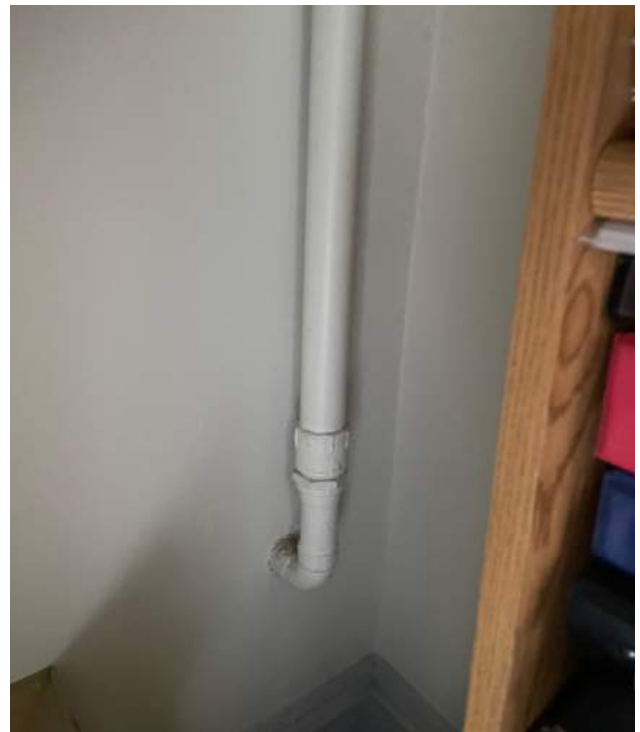
Exhaust pipe in closet.
