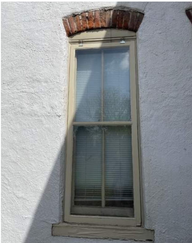
Wood window, storm, and sill on. Brick arched lintel with face brick delamination.
