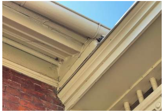
Connection between porch roof and front gable roof.
