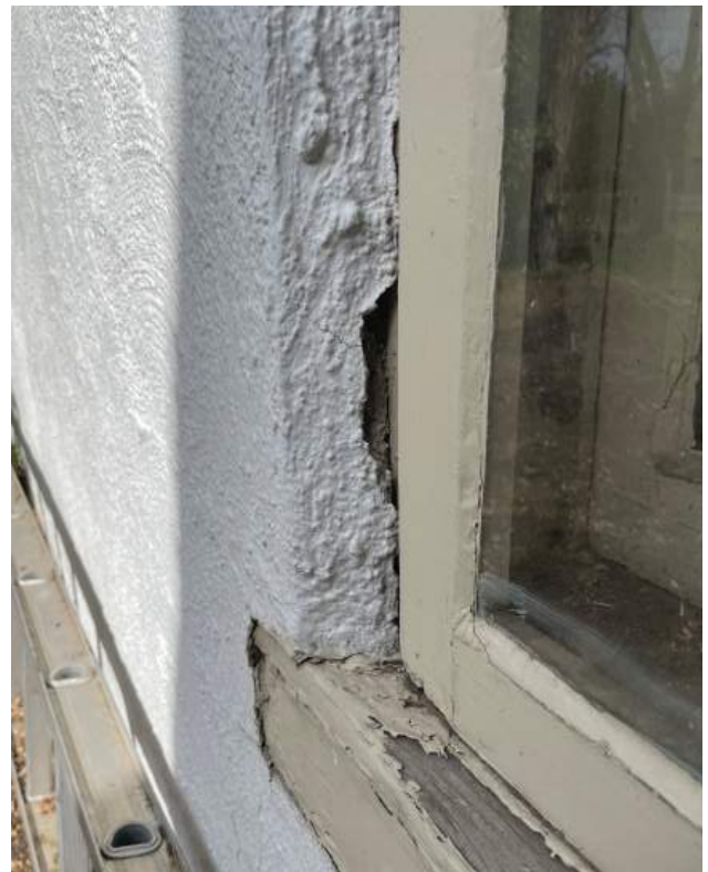
Wood sill paint delamination from water infiltration. Stucco damage at the window jamb.
