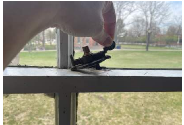
Broken hardware at meeting rail of existing window.
