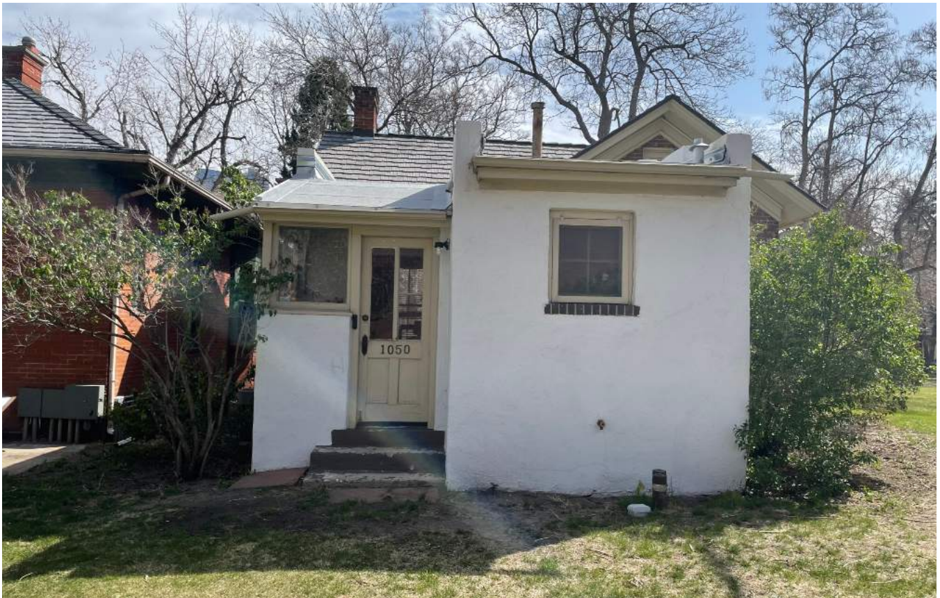
West elevation, stucco finish, wood windows and doors.
