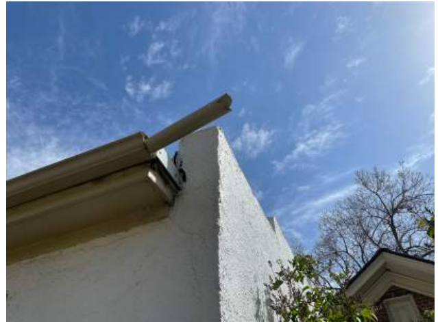
A downspout is missing from the gutter at the west elevation.
