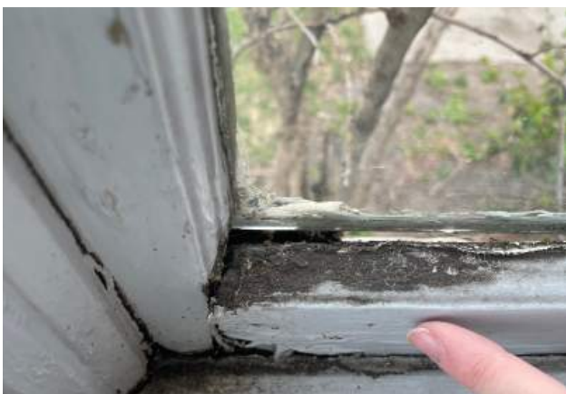
Deterioration at the window frame.
