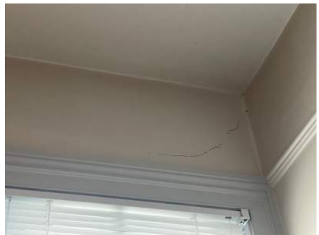
Plaster crack above west facing window.
