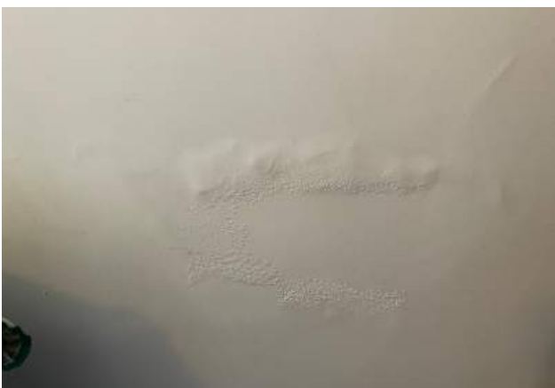
Plaster damage at south wall of existing Office 2.
