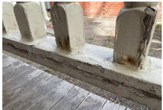
Deterioration of the wood balusters at the porch guardrail.
