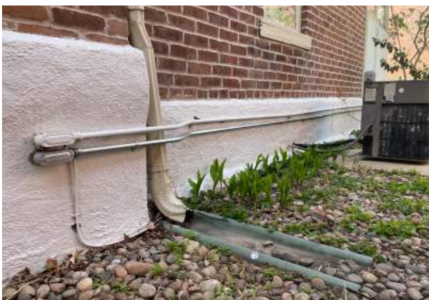
Downspout with splash pad and conduit along foundation wall.
