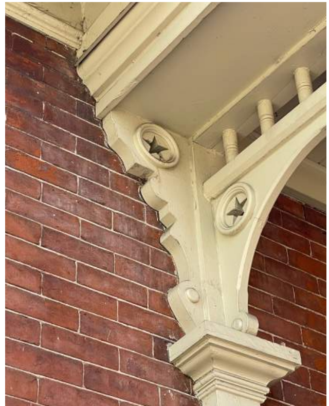
Bracket detail below porch roof.
