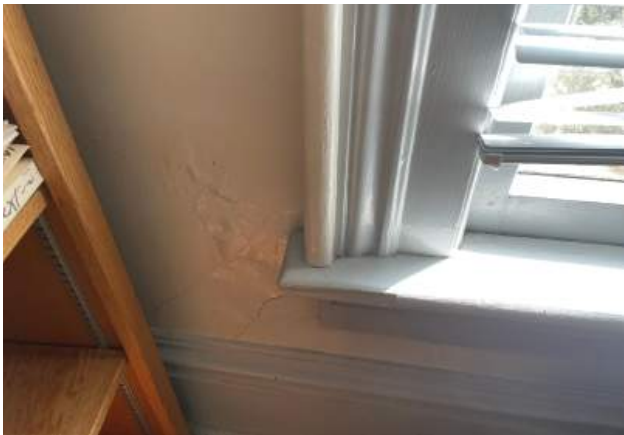
Interior casing and wood stool. Paint bubbling evidence of water intrusion.
