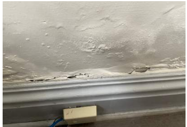
Plaster and paint damage at base of south wall.
