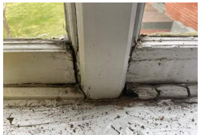
Water damage at the window mullion.
