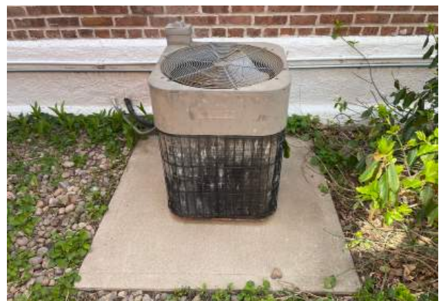
Air conditioning unit on a concrete pad.
