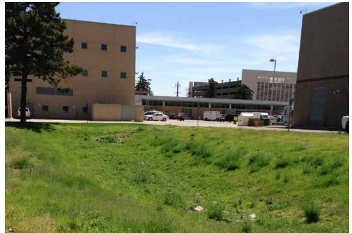
Retention pond north of CUP as seen from 19th Place and Victor Street.
