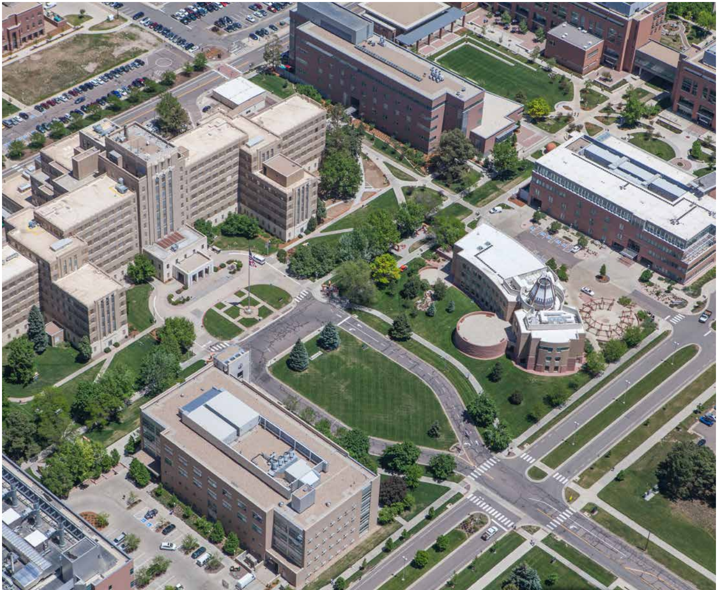
Building 500 (upper left) and forecourt at Aurora Court.
