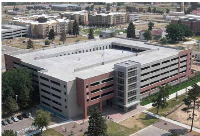
Henderson Parking Garage.
