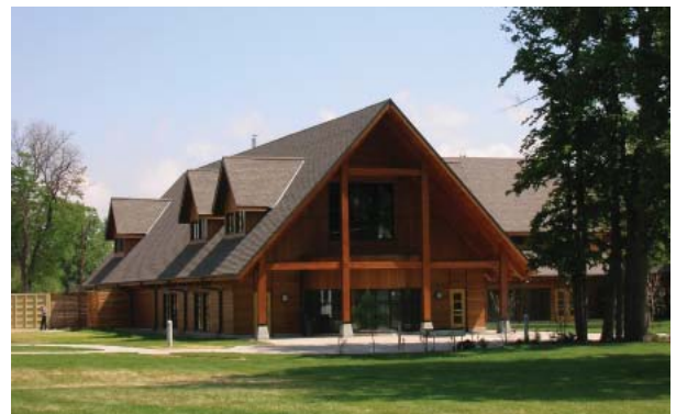
CeDAR's main treatment facility
