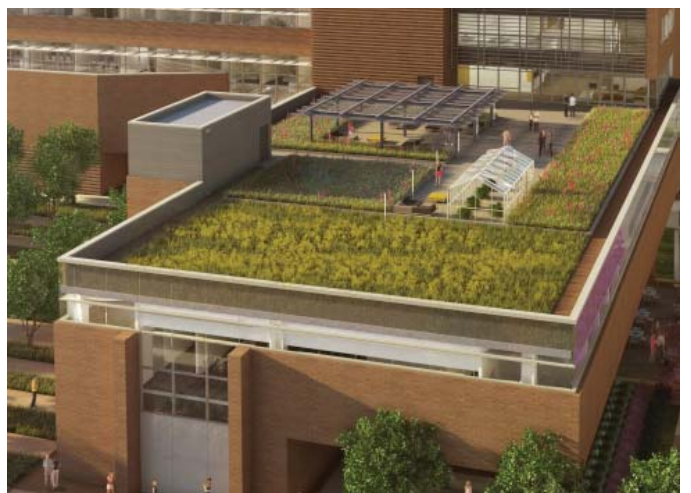
Anschutz Health and Wellness Center - Green roof garden.
