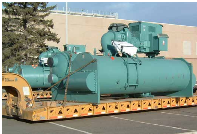
A chiller outside the CUP is about to be installed.
