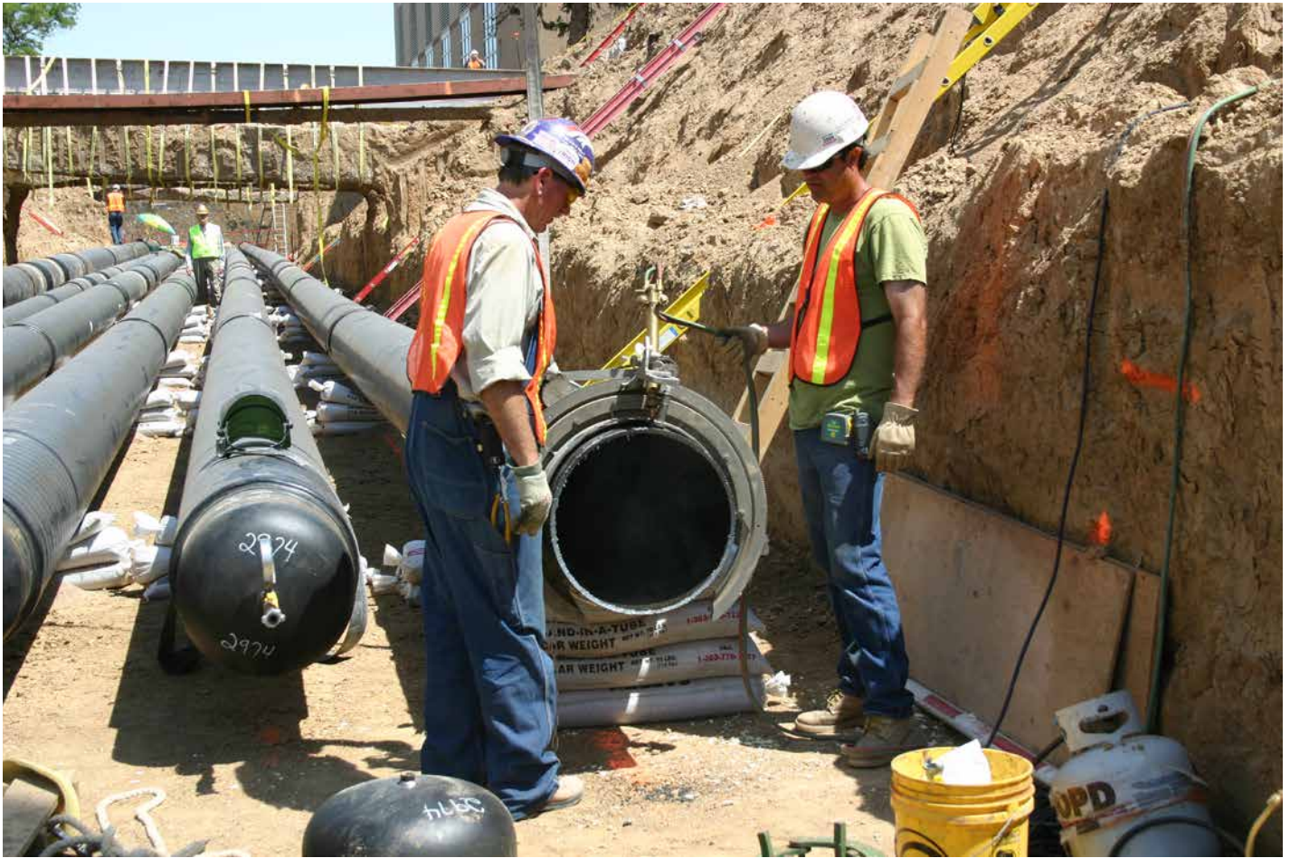
Pipe installation south of the CUP.
