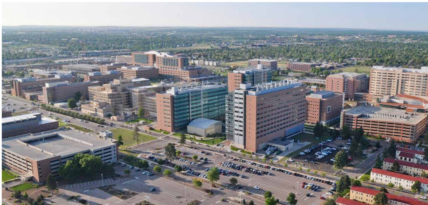
This aerial photograph shows surface parking lots flanked by the Henderson (left) and Leprino (right) parking garages.
