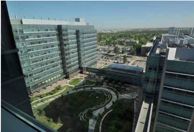
The vivarium expansion is slated to be designed underground, below the northern half of the Research Commons.
