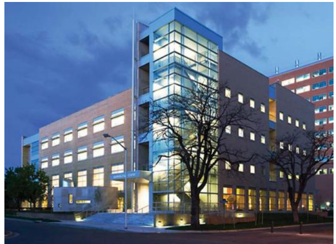
The Barbara Davis Center for Childhood Diabetes, while a predominately clinical use building, was designed with the ability to accommodate future wet-lab research.
