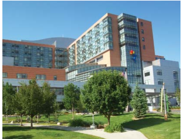
CHCo's Main Tower - "Building in a Park"
