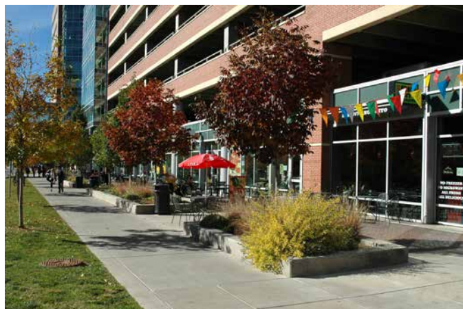
The Leprino Garage on 17th Avenue boasts first-floor retail uses as well as 1,410 parking spaces.
