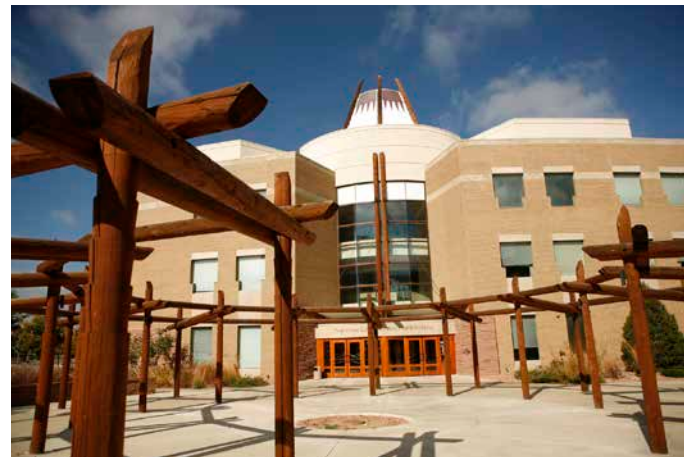
The Nighthorse Campbell Native Health Building was built in 2002 and supports educational, office, and clinical uses.
