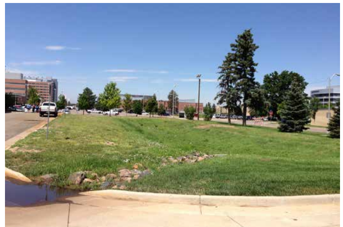
Retention pond north of CUP looking west from Campus Services.
