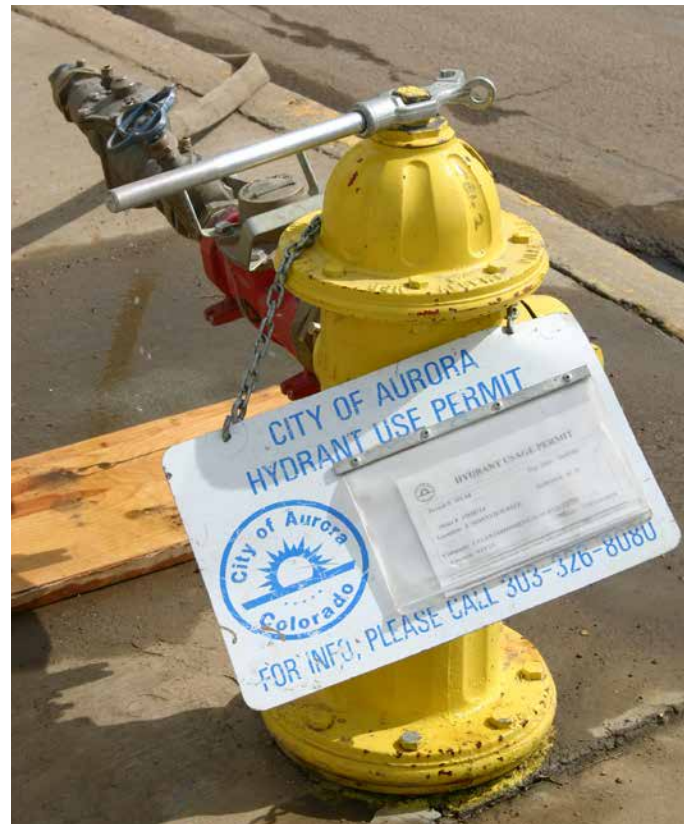
Future development will require upgrading water infrastructure.
