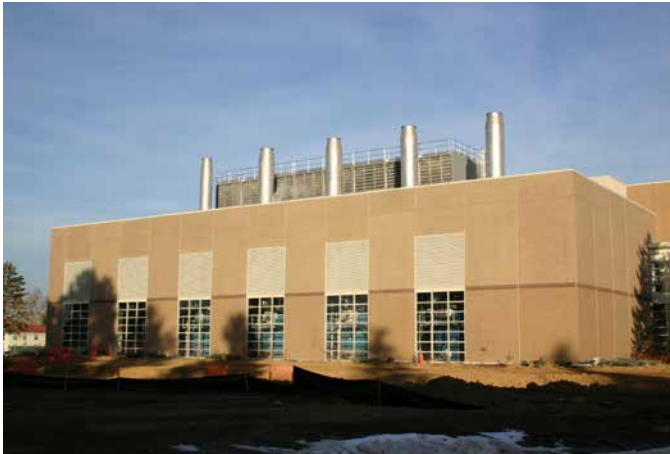
Central Utility Plant.
